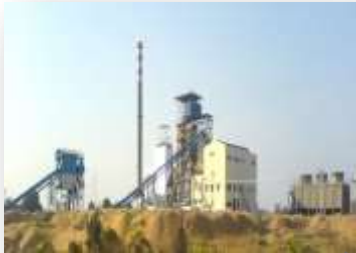
10 MW POWER PLANT FOR VARUN BIO ENERGY
