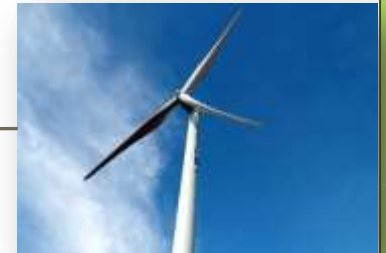
1.5 MW WIND TURBINE AT UTHUMALAI
