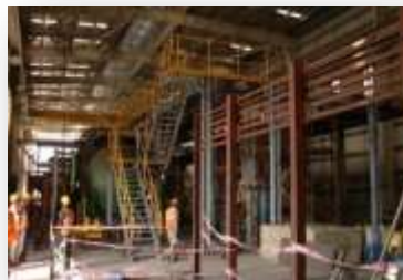
COLOUR COATING LINE FOR TATA BLUESCOPE LTD.
